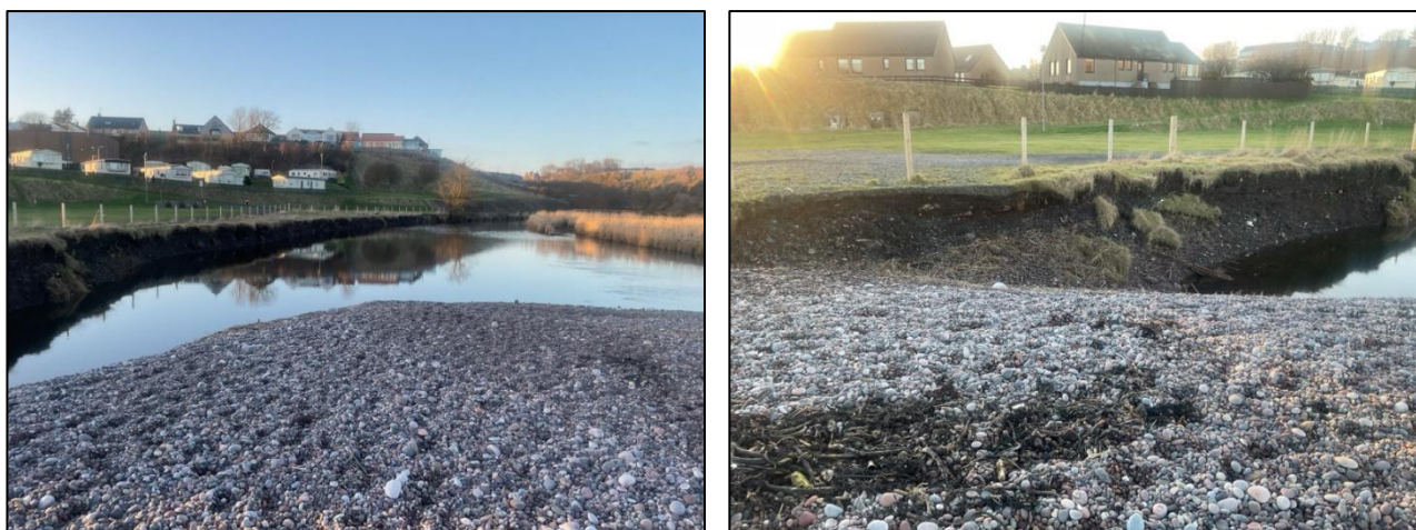
Figure 2-3: Inverbervie Caravan Park boundary and Bervie Water right bank erosion.
